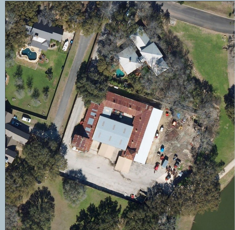
Example of Maintenance Facility
