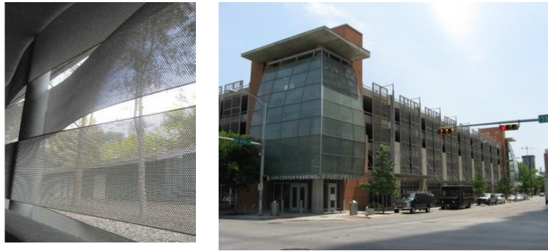
Figures 7-13 Illustrative Examples of Parking Garage Screening
