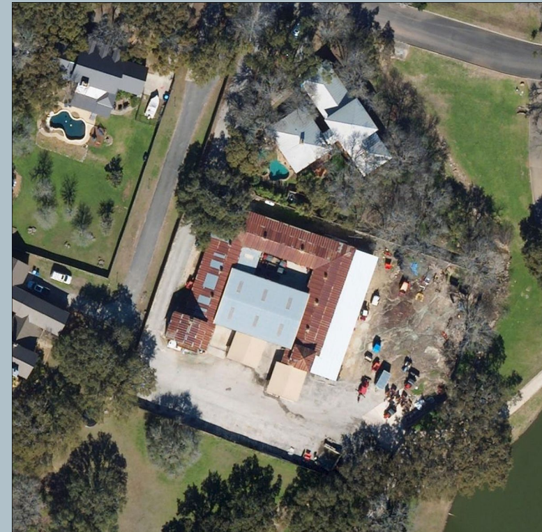
Example of Maintenance Facility
