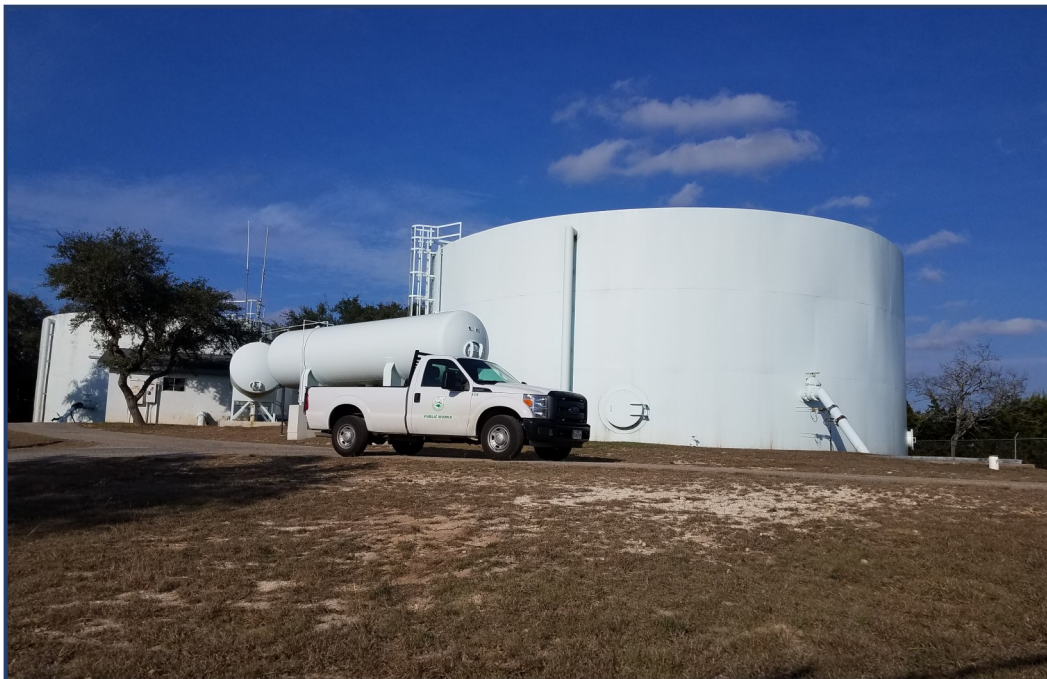
Elmo Davis Water Treatment Plant
