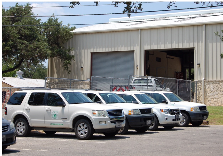
Public Works and Maintenance Building
