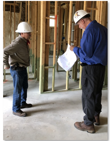
Inspection in Progress
