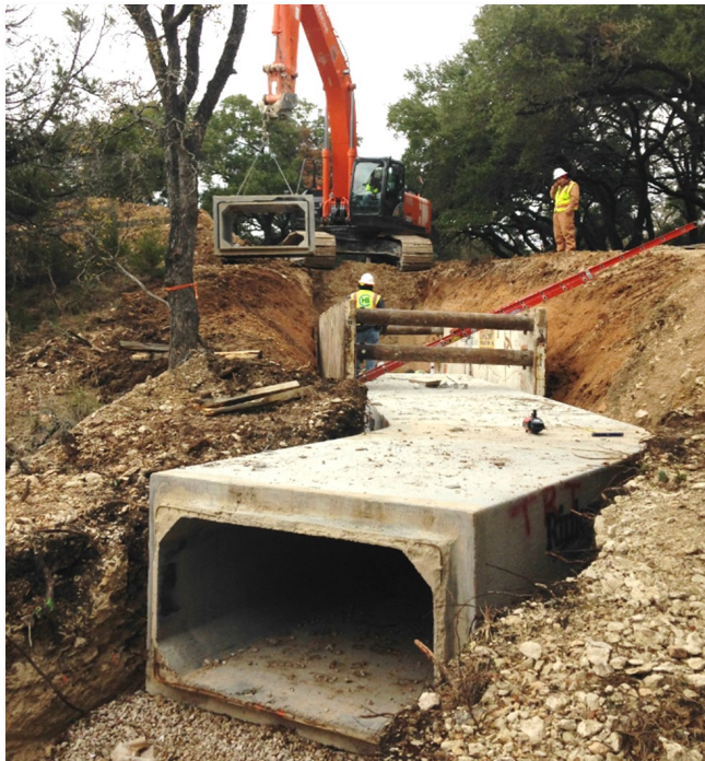
Drainage Project in Progress
