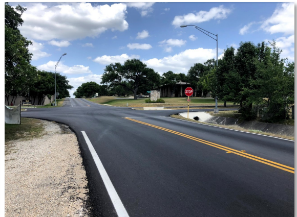
Completed Roadway-Dietz Elkhorn
