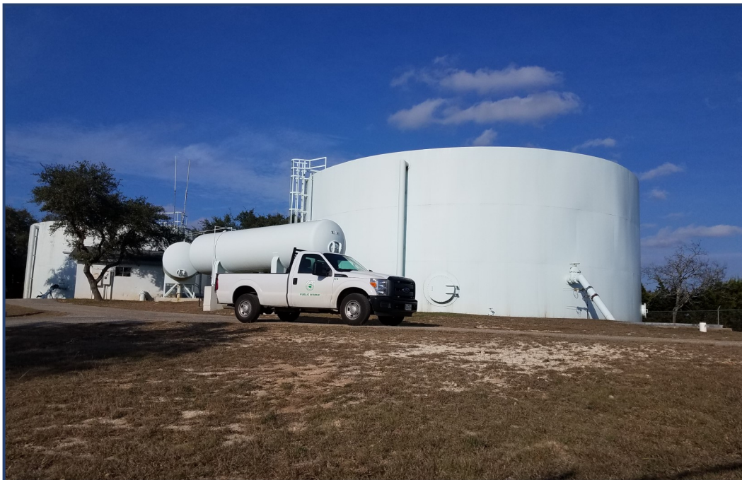
Elmo Davis Water Treatment Plant
