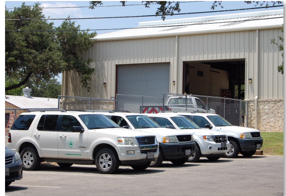
Public Works and Maintenance Building
