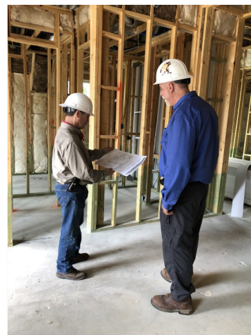
Inspection in Progress
