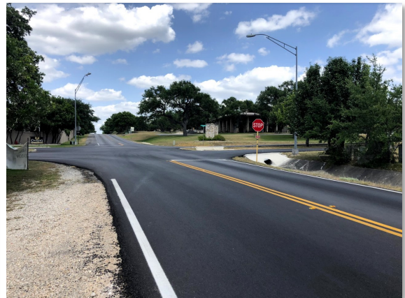
Completed Roadway-Dietz Elkhorn
